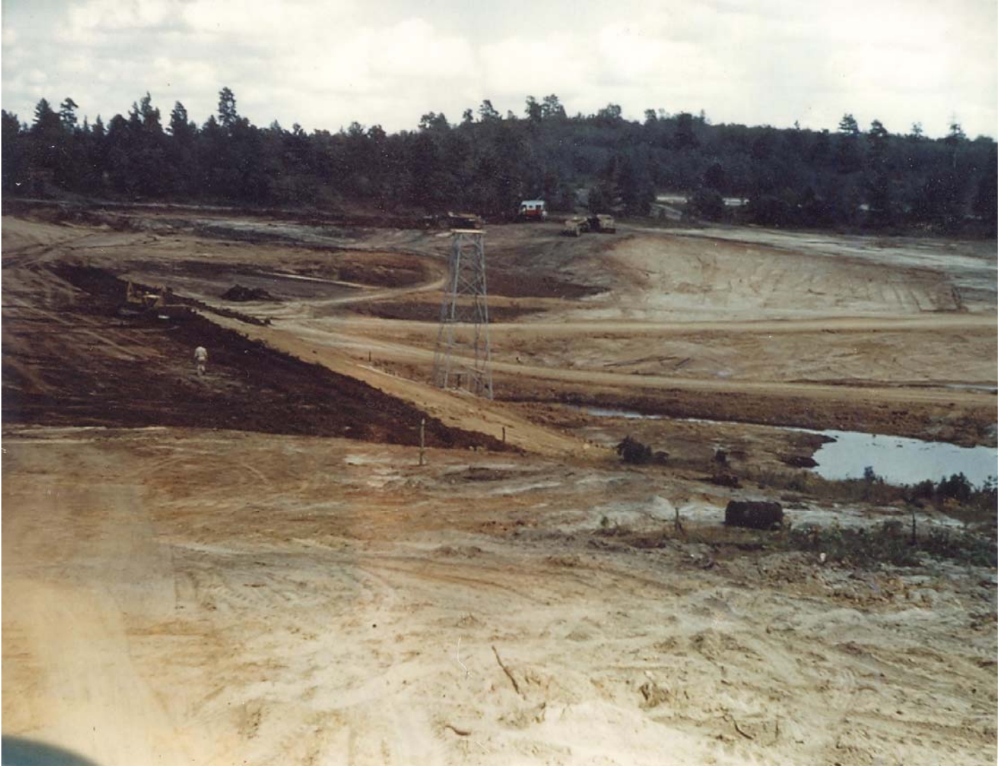
Figure 11. View of what would become Hodges Lake as it was being constructed in the 1950s. Image courtesy of the Hodges Gardens Archives.
