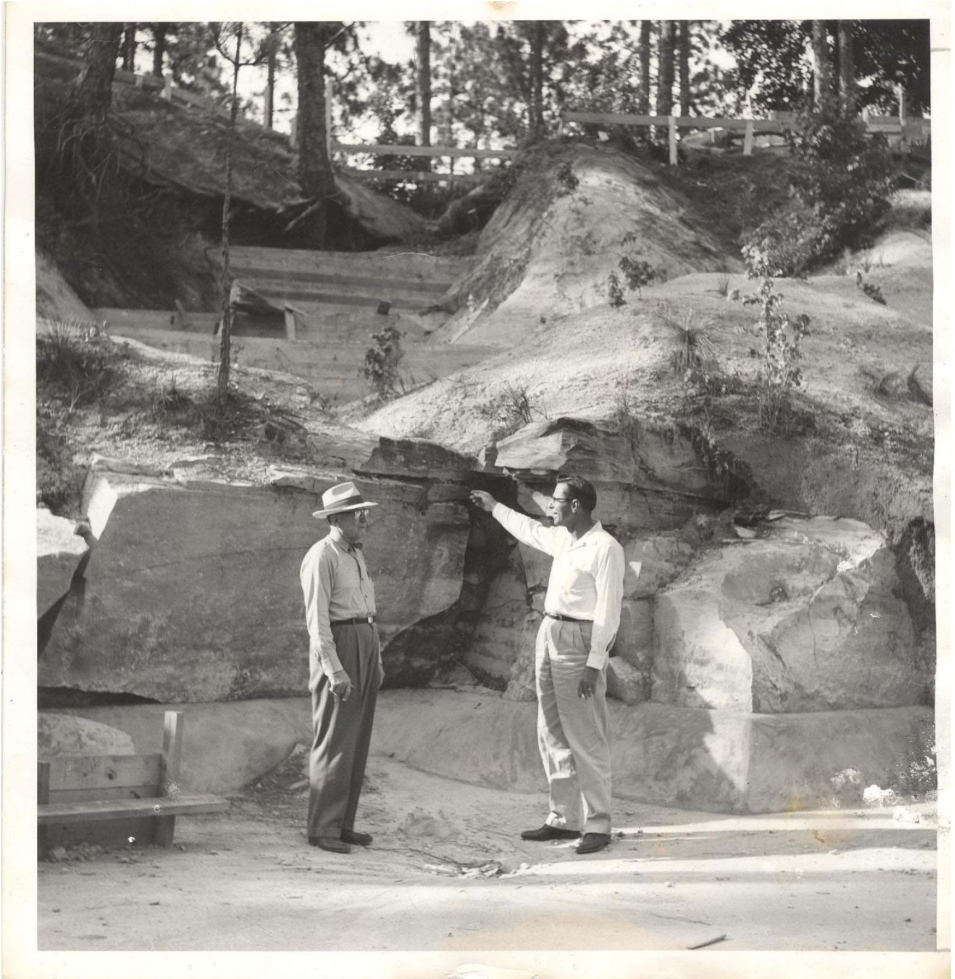
Figure 4. A.J. Hodges and a worker discussing plans during the gardens' construction (notice the original quarry in the background). Image courtesy of the Hodges Gardens Archives.
